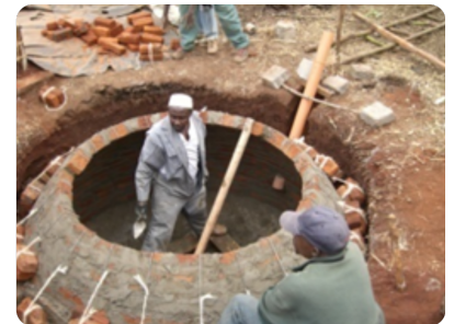
Construction of biogas units for households in Kenya
